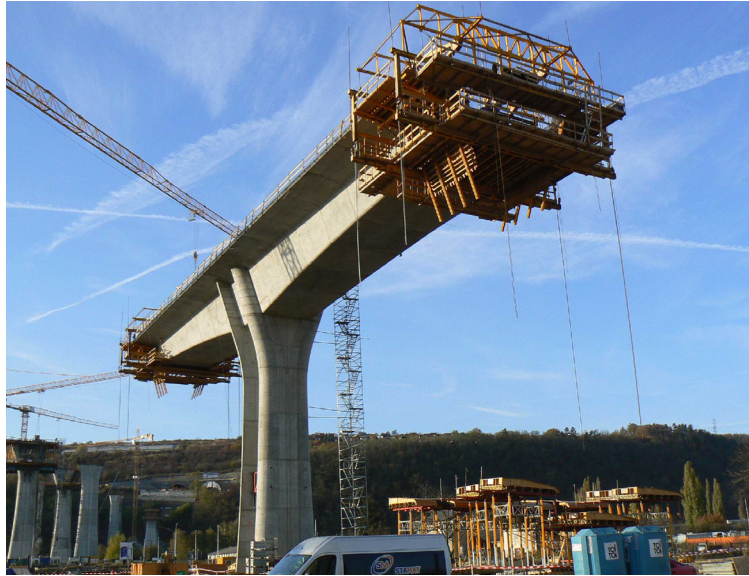
Figure 34: Construction process of box girder bridge
