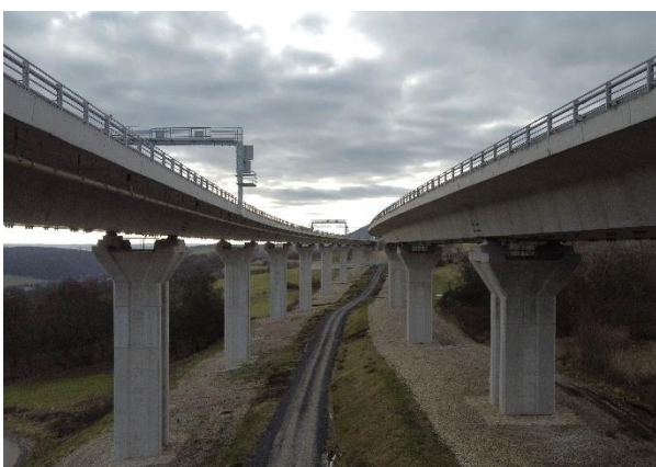
Figure 8. A view of the investigated viaduct.
